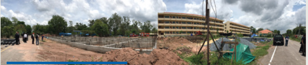
Construction of the warehouse is underway in Thailand.
