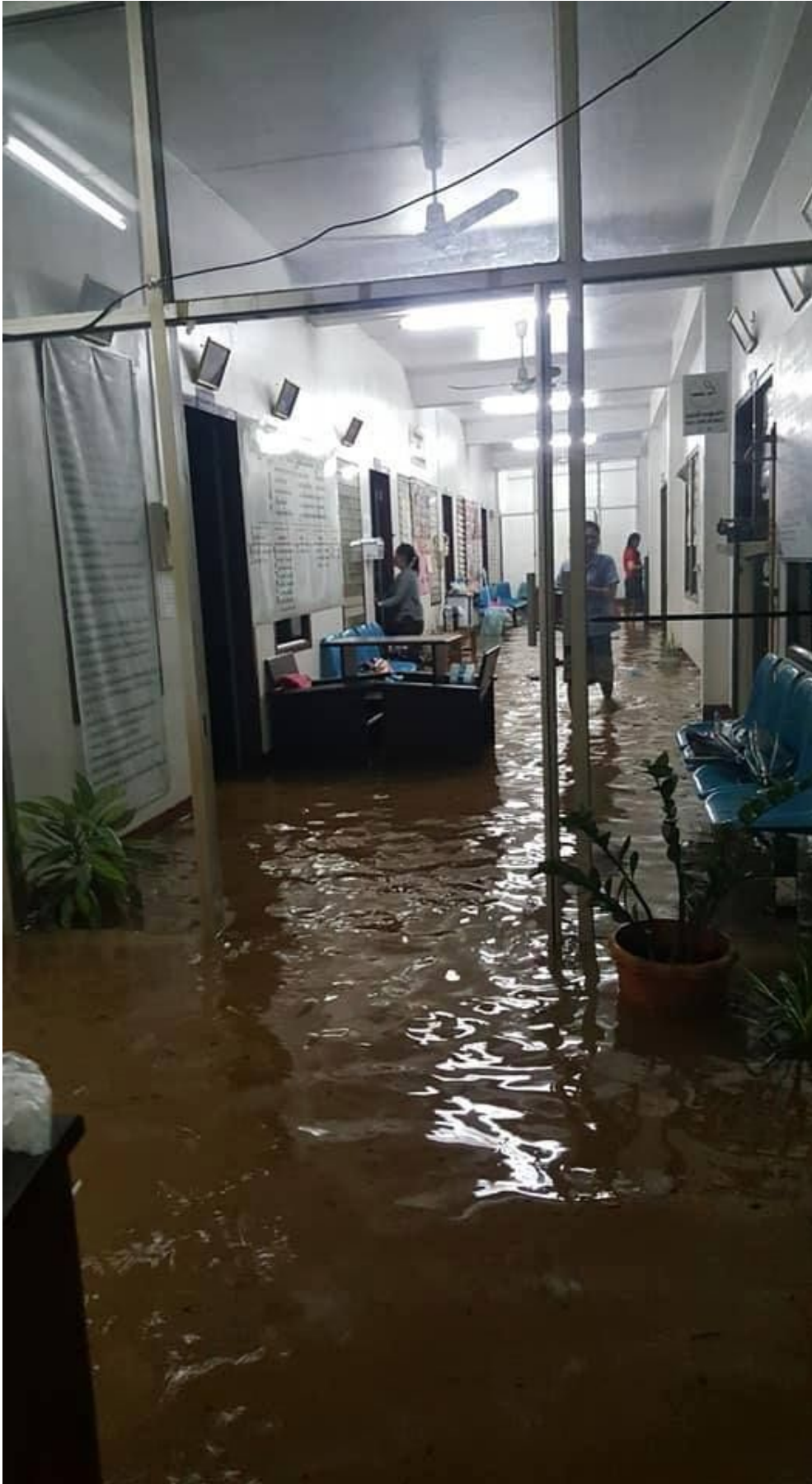
Figure 8: Champasak provincial hospital completely inundated
