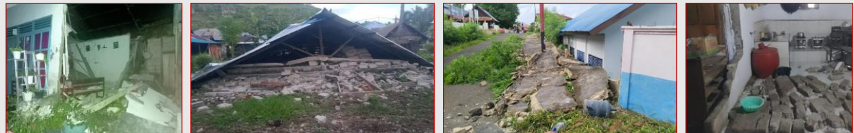
Reported damages in the affected areas (Source: BNPB )
