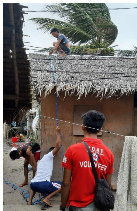
Figure 6.9 Installing SSKs in Camarines Norte (source: PRC).
